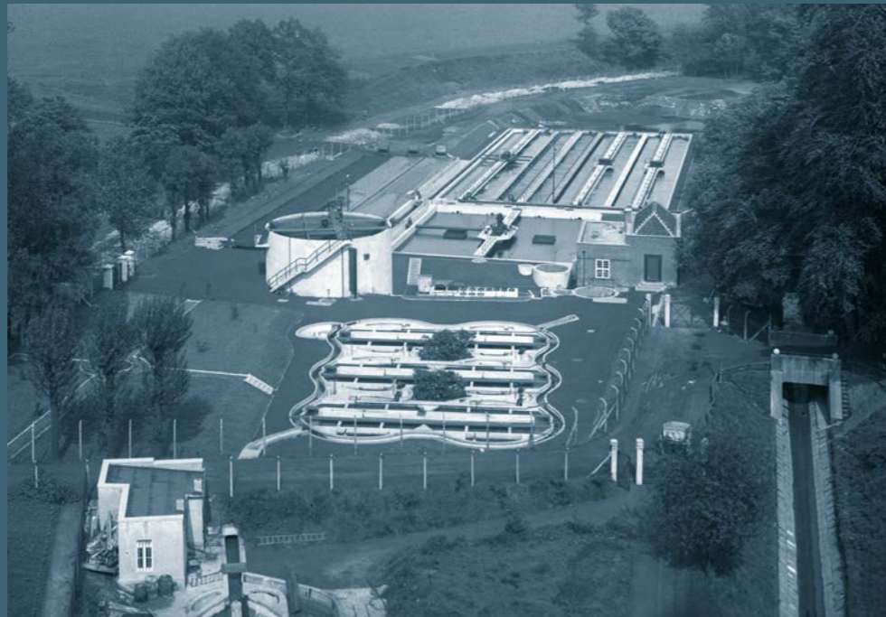
Waste Water Treatment Plant Essen-Rellinghausen, the first operational German waste water treatment plant using the activated sludge process
