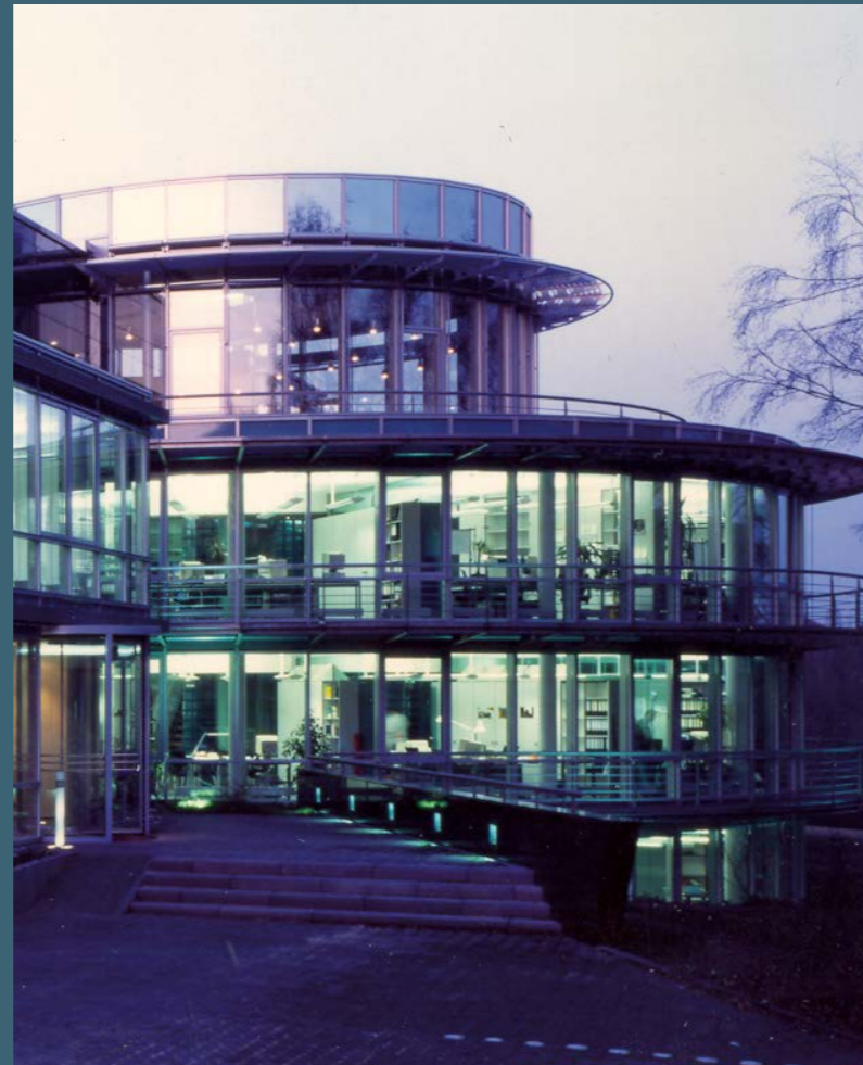
The engineering company DAHLEM moves into its own premises
