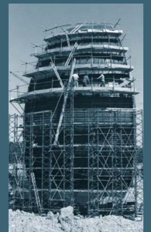
WWTP Münster, Digester in segmental construction
